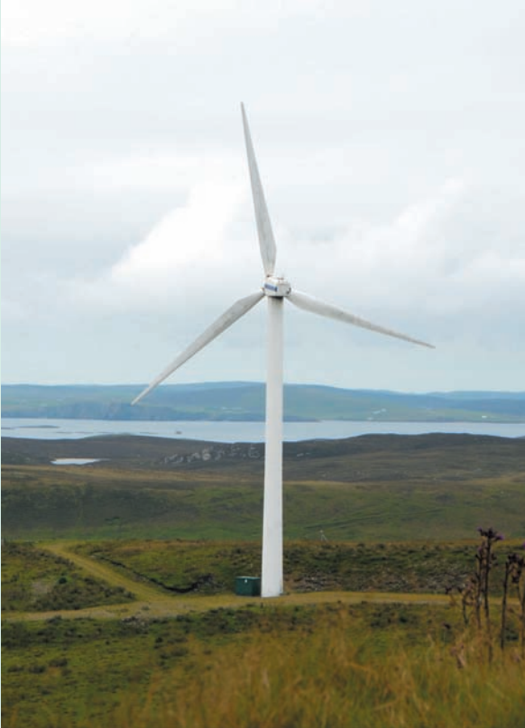
In 2012, this was just one of the five windmills generating electricity on Shetland. But all this was about to change if the new proposals were approved by the Scottish Government.
